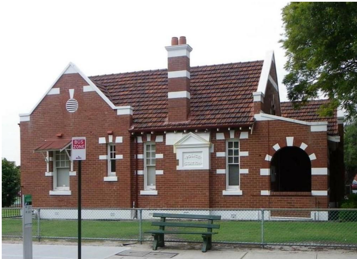
Labouchere Road façade of the South Perth Police Station and Quarters (Former) . (Gina Fraser, City of South Perth, 2015)
