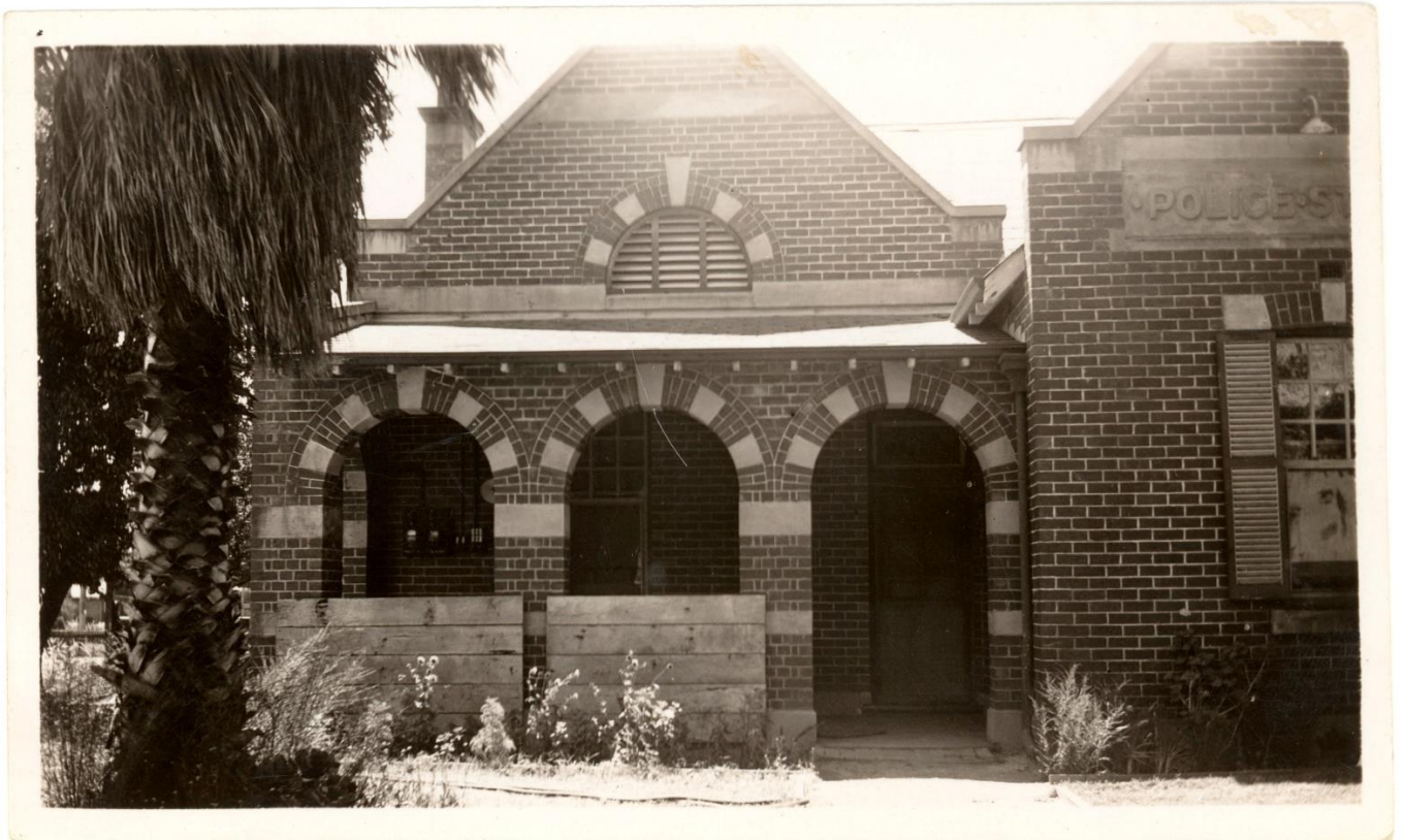
South Perth Police Station and Living Quarters (Former), view from Mends Street. Courtesy of WA Police Force Records and Management Centre, Perth.
