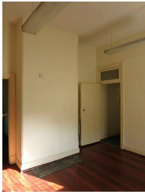
View across former charge room towards door to cells (right). A former fireplace bricked up (centre). Doorway to living quarters on left.
